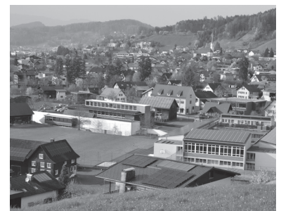
Photovoltaikanlagen in Muntlix
